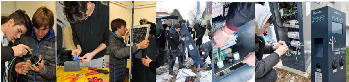
Picture 3: Equipment installation and charging station set up (Photo: S. Simović)
