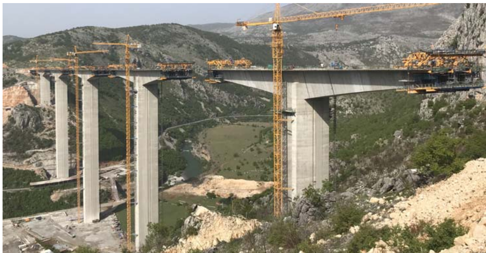
Figure 1: Realized part of the bridge construction as of 25. 04. 2019.
