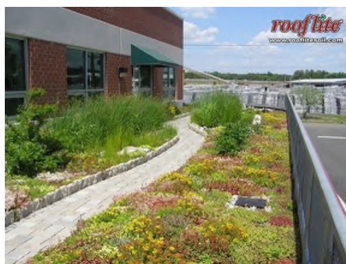
Picture 2: Semi-intensive green roof
