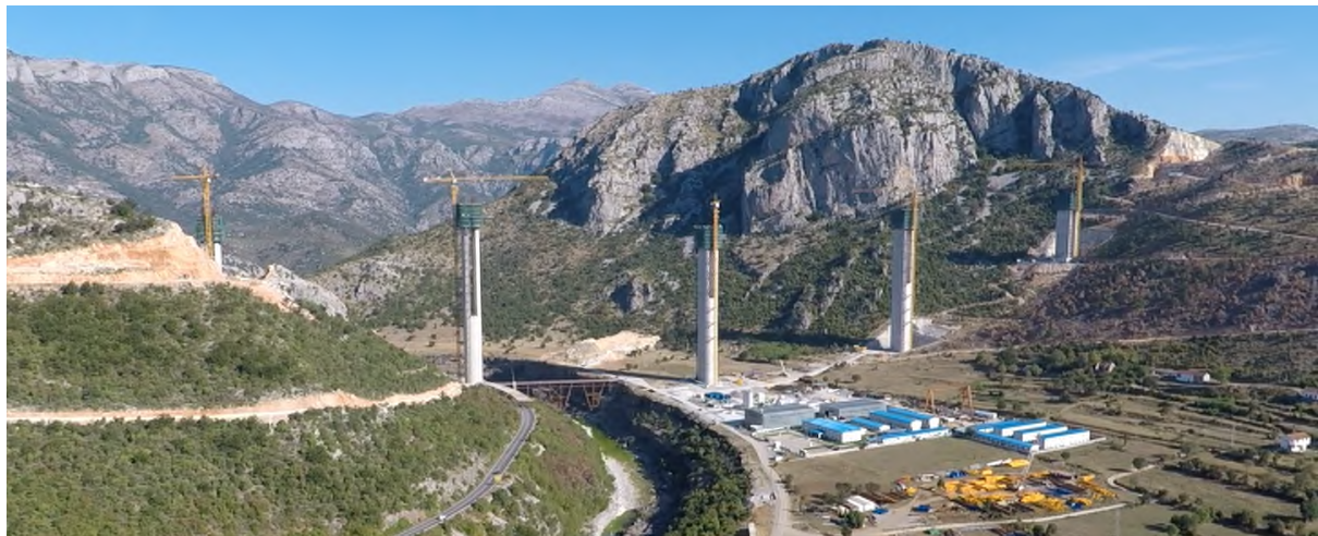
Figure 1: Realized part of the bridge construction as of 15.09.2017.
