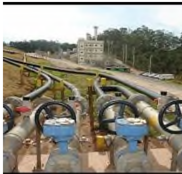
Figure 3: Gas distributor
