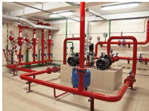
Figure 4. Sprinkler station
