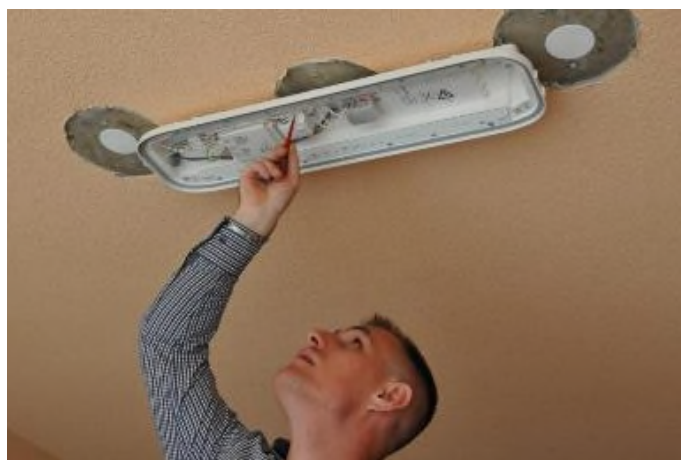
Picture 3: Installation of new lamps FORCELED 4000 HF L840
